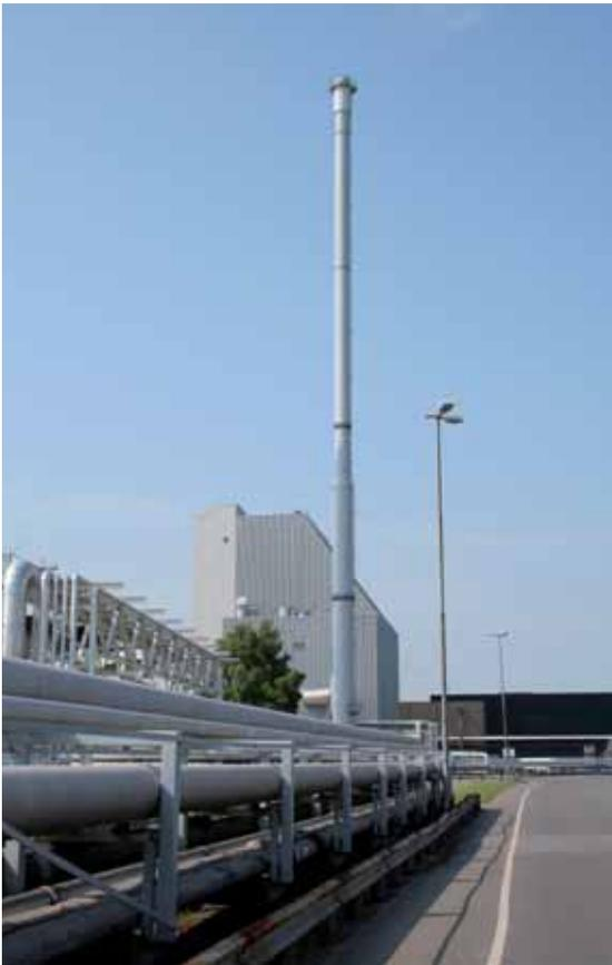
More than two thirds of Borregaard's energy consumption is thermal energy, mainly in the form of steam. The biomass boiler that was opened in 2005 utilises waste from production to produce heat.
